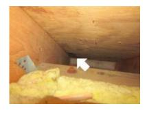
Roof Support: Some truss members have been cut to accommodate the installation of the air
